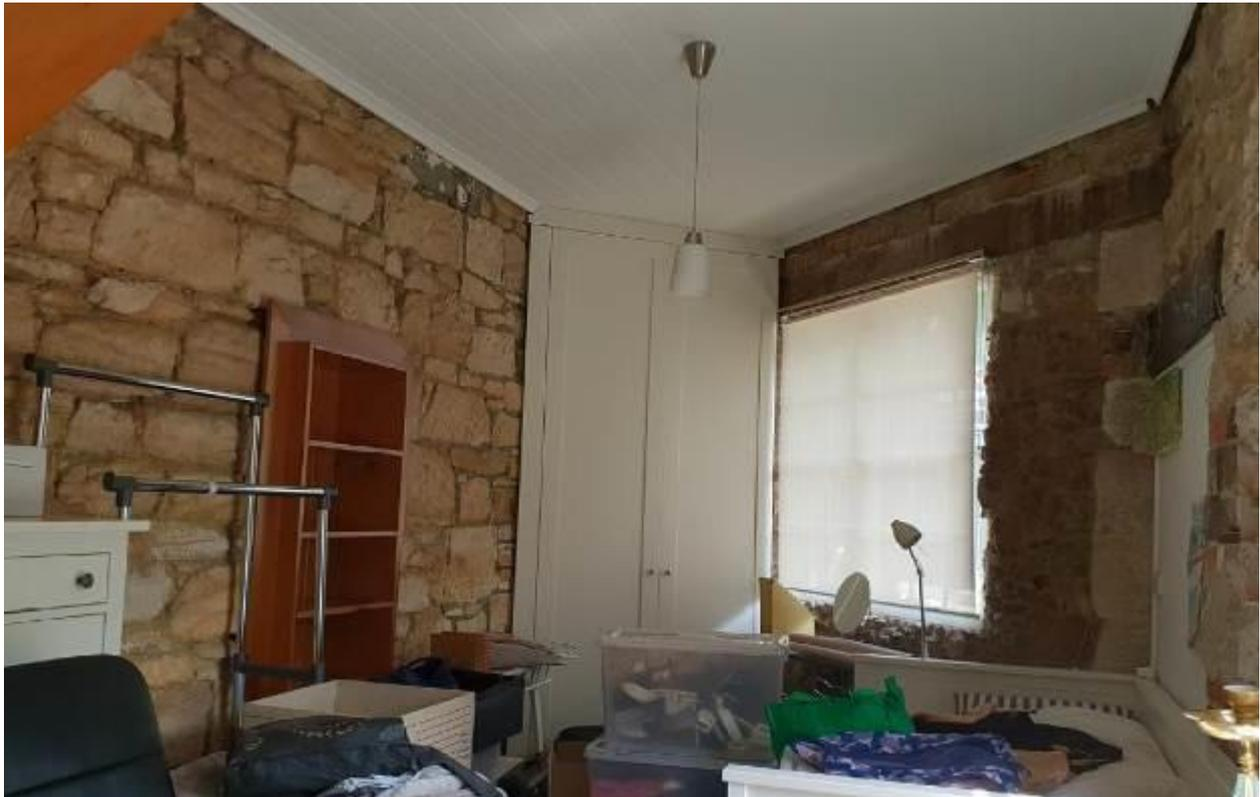
**Figure 4: views of the front room at ground floor with the previous link to no.59 (bookshelf), the infilled front shopwindow and the entrance door to the right.**
